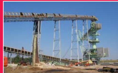
A-frame structural support bents support a trussed conveyor feeding a raw material storage pile.
