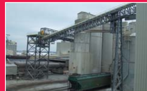
A trussed Rapat conveyor and transfer tower are shown moving limestone at a processing facility.
